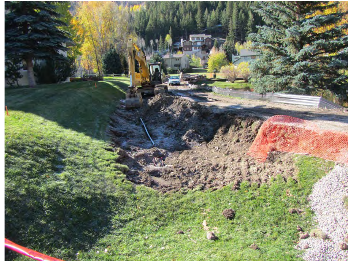
Flood Bypass Channel enlargement during Construction
